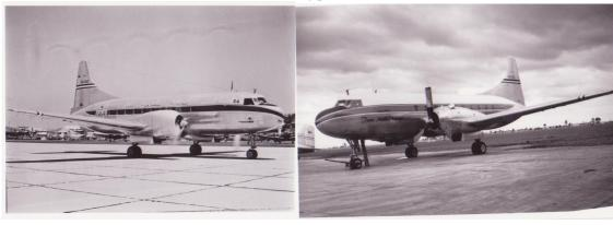
The one on the left is VH-TAQ on the tarmac at San Diego, all bright and highly polished and the second photo is in Melbourne after it was decided that the upper part was to be painted white to reflect the sun and reduce the heat inside the aircraft during turnaround. Note where the name *Trans-Australia Airlines* was painted on the initial aircraft, and it was later repositioned along the fuselage and above the windows.
