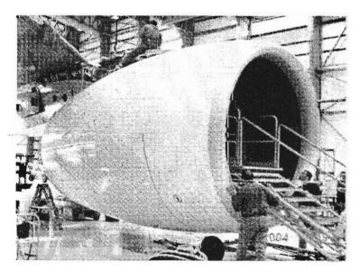
Just to show how big the aircraft and engines will be, this photograph shows the size of the inboard (No.2) engine being fitted at station 30 – note the Engineer guiding the engine onto the pylon, with minor adjustments being undertaken by two engineers at the front of the engine. I was unable to establish the weight of the engine but expect it to be in the vicinity of 20 tonnes.
